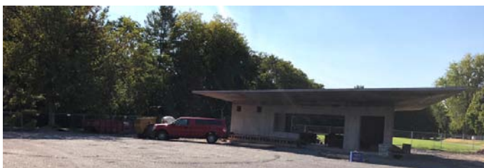
The field house construction in progress, September 24, 2018.
